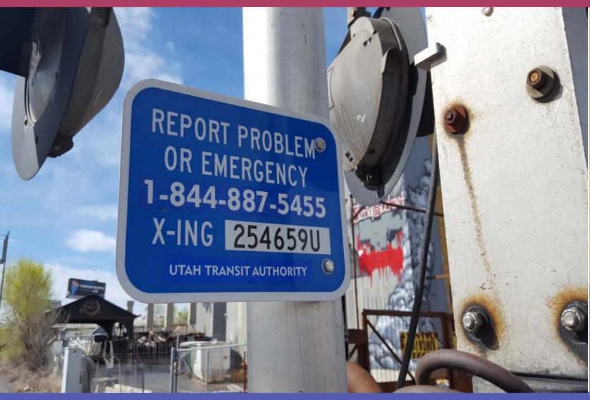
It is used to notify the railroad of an emergency or warning device malfunction.
