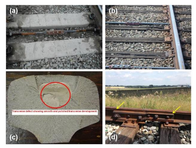
Figure 3 – Typical track and tie defects: (a) Cracks at centers of ties at POD (NSTB RAB1411); (b) Deteriorated crossties at accident location (NSTB RAB1606); (c) Transverse defect of rail track (FRA track inspector reference manual 2015); (d) Compromise joint bar (NSTB RAB1409)
