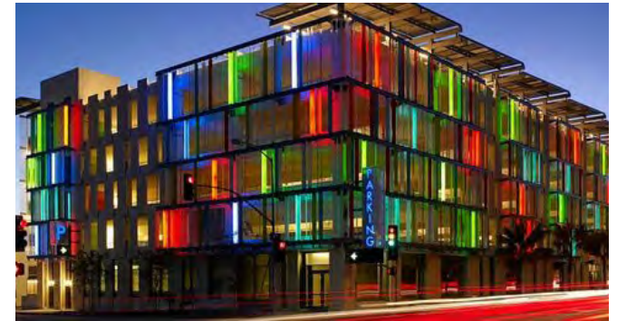
Santa Monica, California Parking Structure
