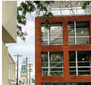
Columbus, Indiana Parking Structure
